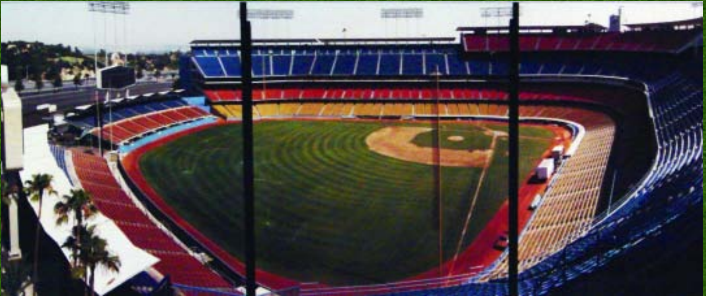
Dodger Stadium, Los Angeles, California Dodger Stadium in Los Angeles was built in 1962, and maintains a status as one of the best places to play and watch a baseball game. An abundance of good weather, fanatical attention to maintenance and detail, and a corporate attitude that suggests it knows it's in the entertainment business, add to the glamour and ambiance. Sandy Koufax played here. Vin Scully announces games here. "Dodger Dogs" are sold here. Hollywood comes here.
